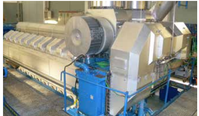
Turbocharger and Heat exchanger
